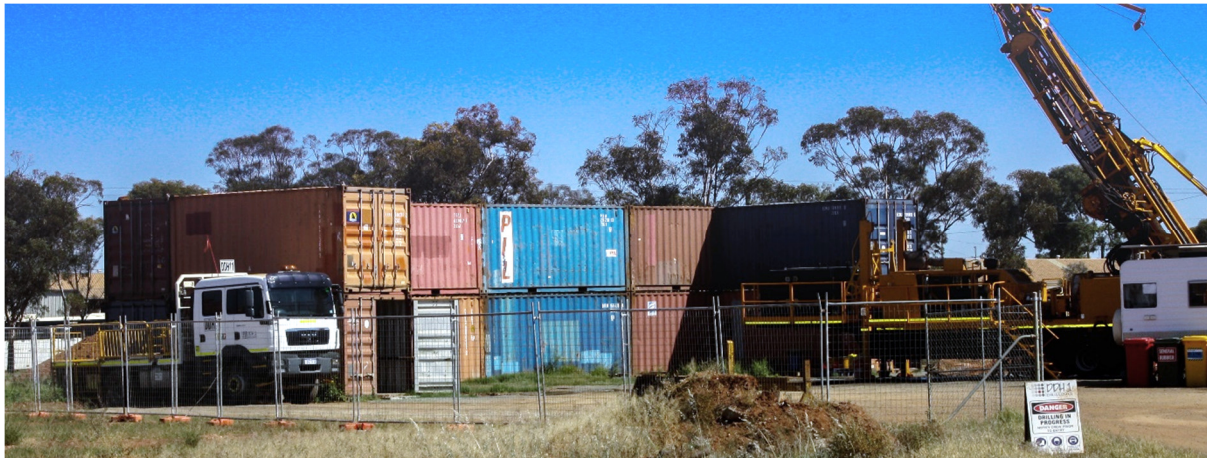
Plate 5-1: Noise barrier to reduce noise from drilling activities at sensitive receptors
