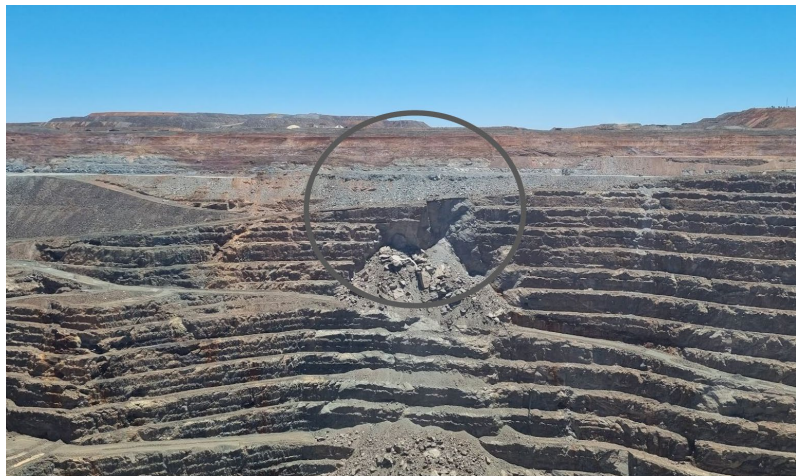
East Wall Slip – May 2018
