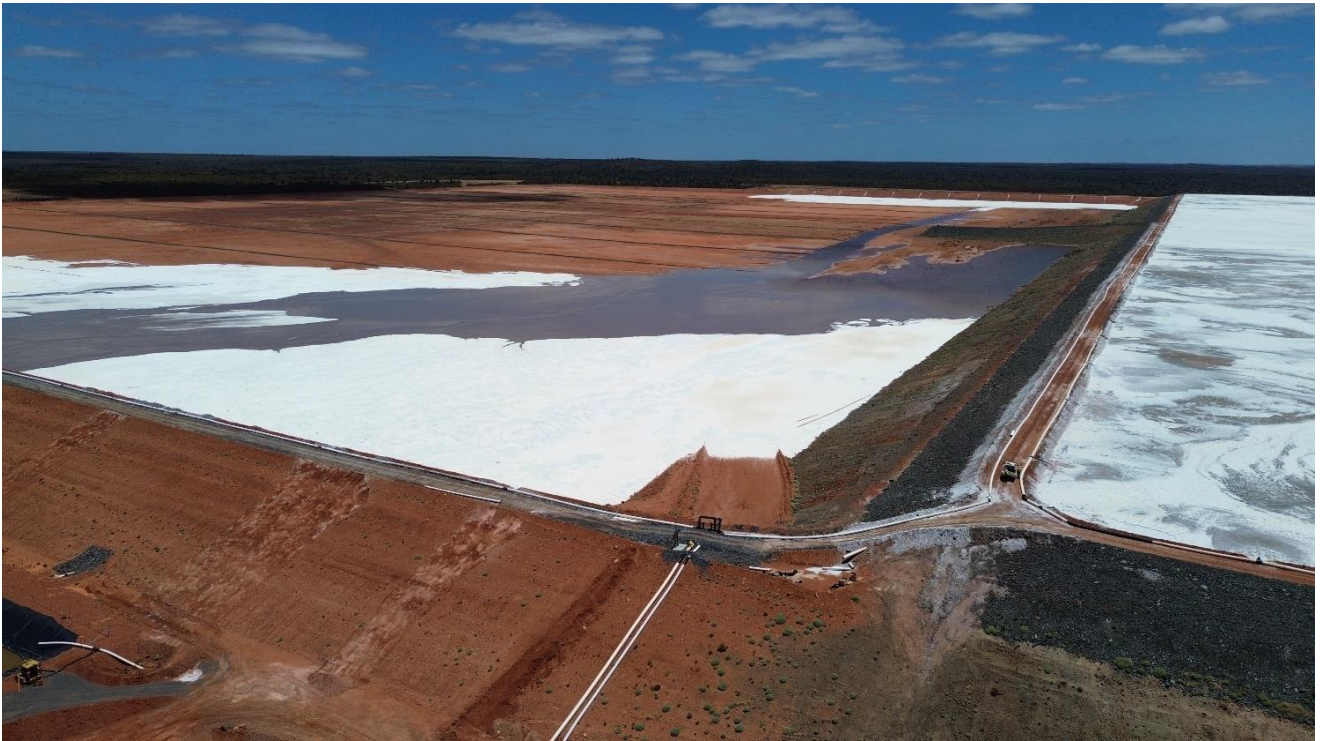
Plate 4 TSF Cell 4 - Commencement of Tailings discharge.
