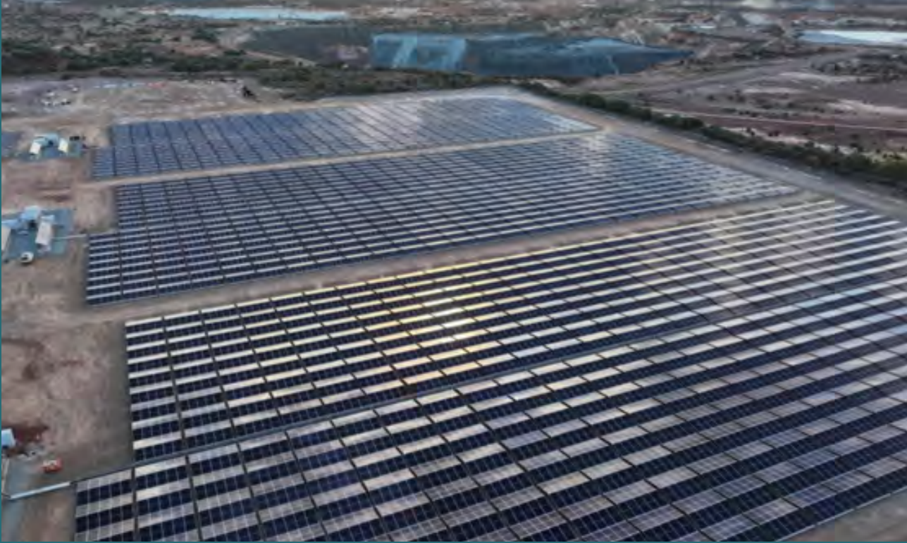
Figure 4 Completed solar farm at Jundee Operations
